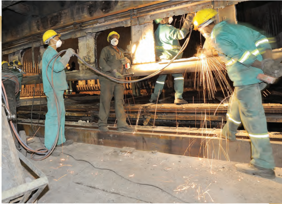
Repair work being done on the boilers of van Eck power station.
