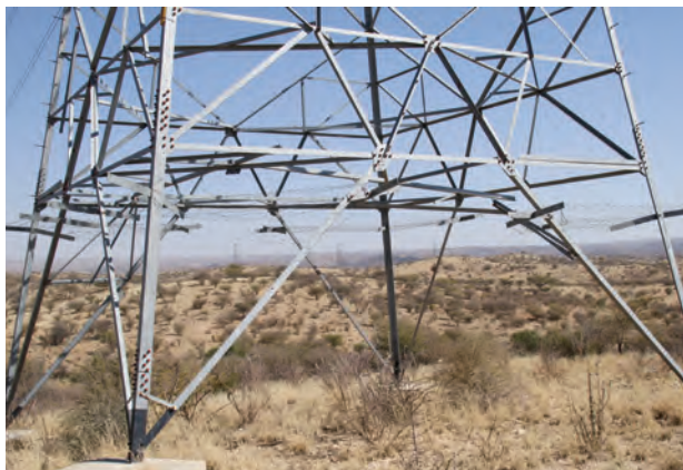
A high voltage power structure without cross braces at the bottom.
